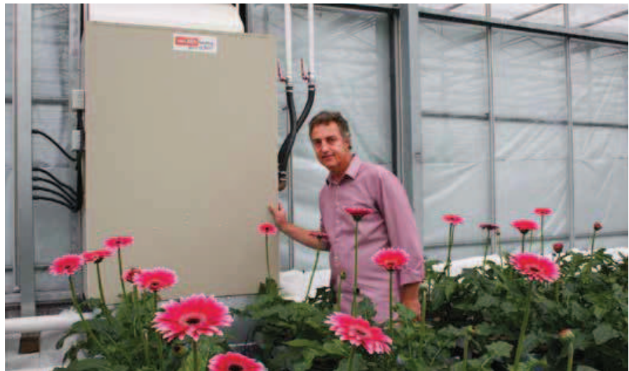
Joek van der Zeeuw: “By using the system to inject outside air into the greenhouse we get a small amount of over pressure. As a result, the temperature distribution throughout the greenhouse is more uniform.”
