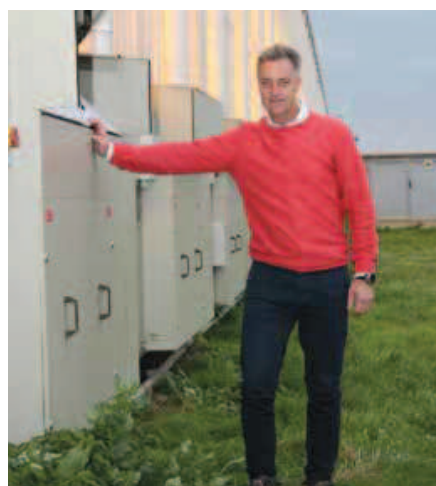
Joek van der Zeeuw “Reducing the height of the AHUs was quite a challenge.”
