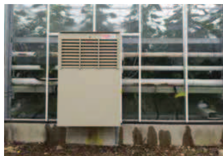
Thirteen units, which are made entirely of plastic, were installed in the two greenhouse blocks at the base of the gable walls.
