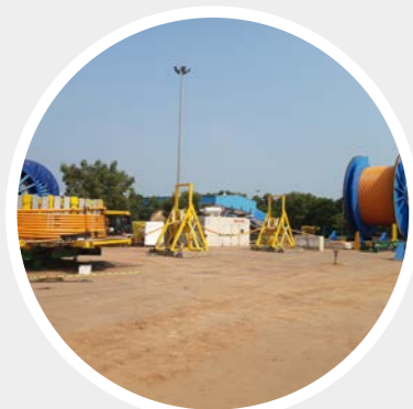
Spooling from reel to pallet/reel & cut to required length
